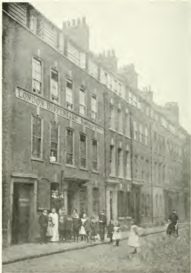
Silk-weavers' Houses in Church Street, Spitalfields (Showing wide attic windows)
